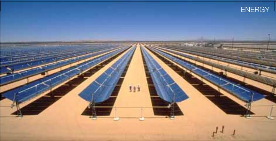
**Figure 4** Parabolic trough concentrating solar collector field of the 150 MW (5 × 30 MW) steam cycle solar electricity generating systems at Kramer Junction, California (Source: KJC)
