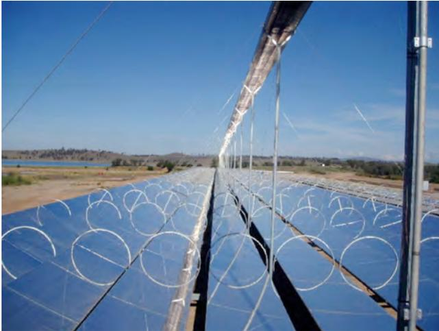
Fig. 1: A recently installed CLFR array segment in Australia. Tracking linear reflectors focus solar energy on elevated boiler tubes to produce steam.
