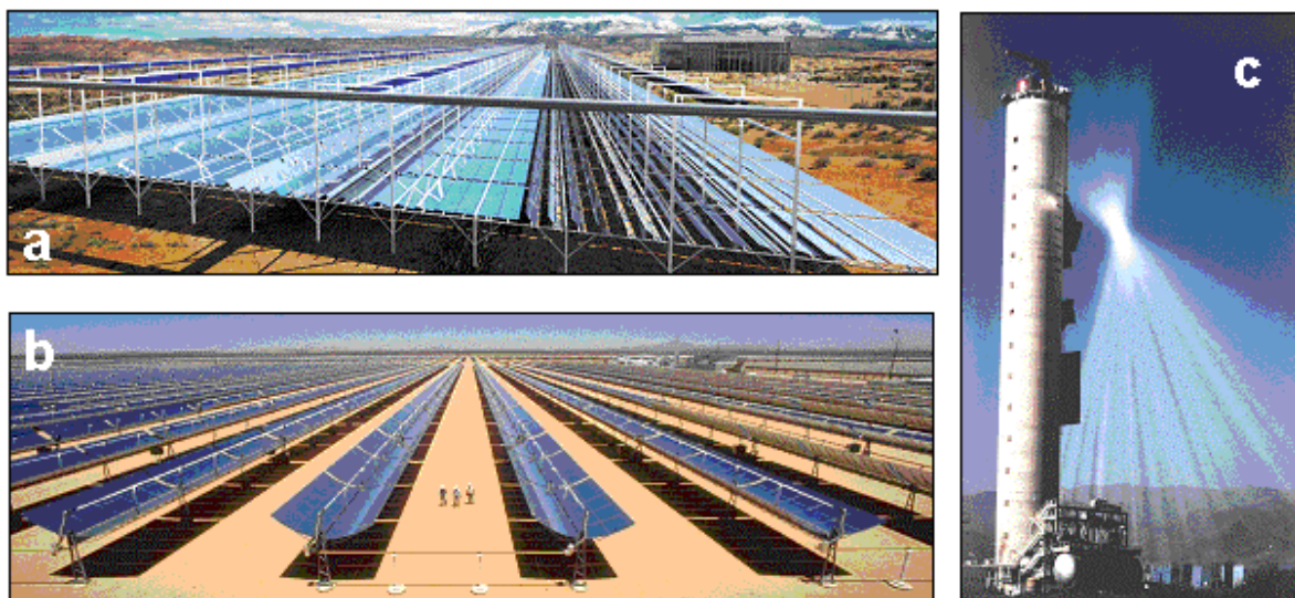
Figure 1: Concentrating solar collector systems with (a) Fresnel concentrators, (b) parabolic trough concentrators and (c) the solar tower concept with surrounding heliostat field.
